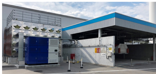
Self-supporting stationary FC generator diverting on-board FC (Shimoyama Plant) Power generation using hydrogen is possible even in power outages
