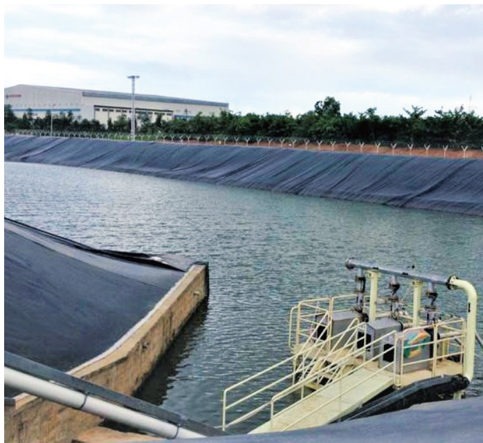
A rainwater reservoir (left) and rainwater treatment equipment (right) at Toyota Kirloskar Motor in India
