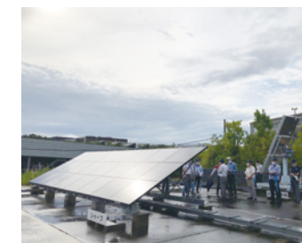
Members of the Kyohokai research groups toured the solar power generation verification site at the Motomachi Plant
