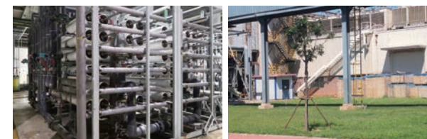
Wastewater recycling production facility
